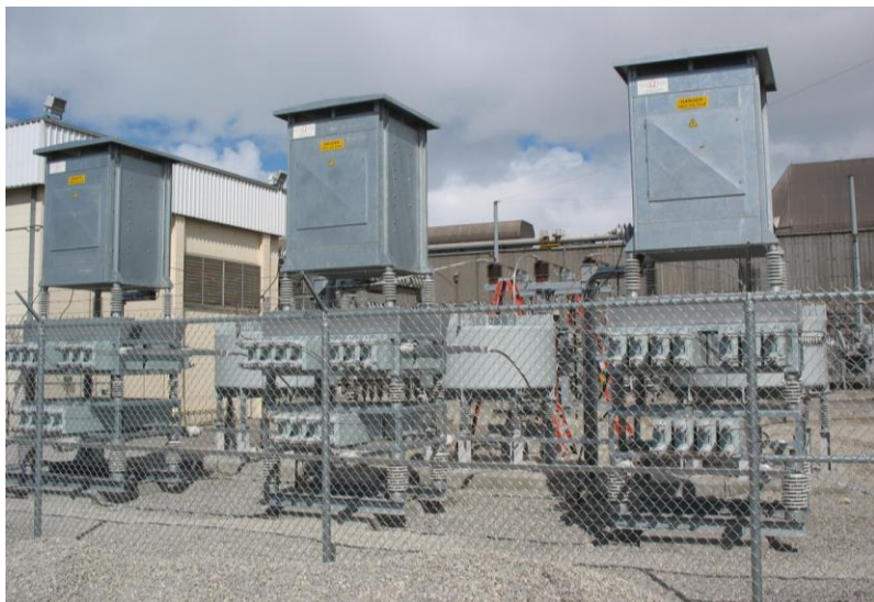
Fig. 5: New 2 nd harmonic filter
