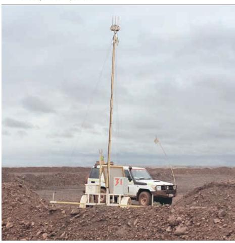
ures. With ABB's solution, high availability and reliability are achieved as Tropos routers operate in a mesh topology with multiple paths through the network, dynamic operating frequencies, multiple radios, and multiple retransmissions on every packet.
