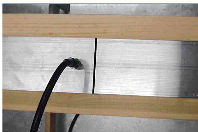
2 Where Waveguide sections are joined, a narrow sleeve is used. This assures galvanic isolation without any degradation of transmission.
