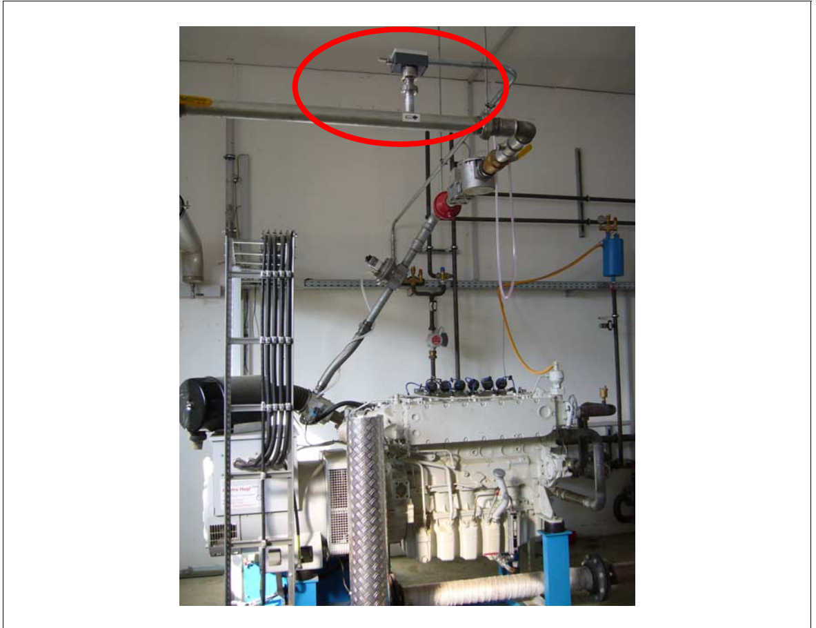
Fig. 2-2: Thermal mass flowmeter in the biogas pipe upstream the block heat and power plant with gas engine
