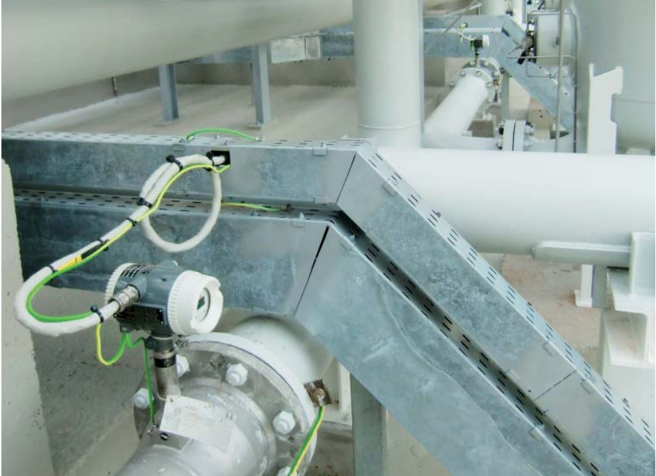
8" (DN200) swirl flowmeter with low space requirements
