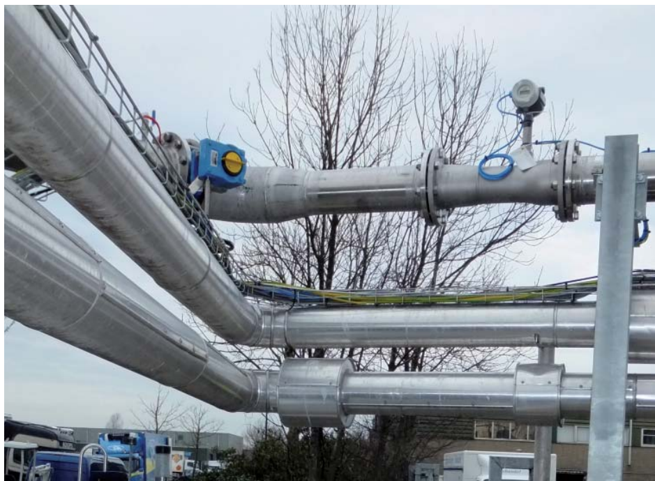
6" (DN150) swirl flowmeter in outdoors biogas application
