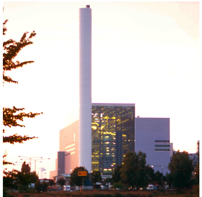
Fig. 6: Stack with many upstream straight stack diameters available
