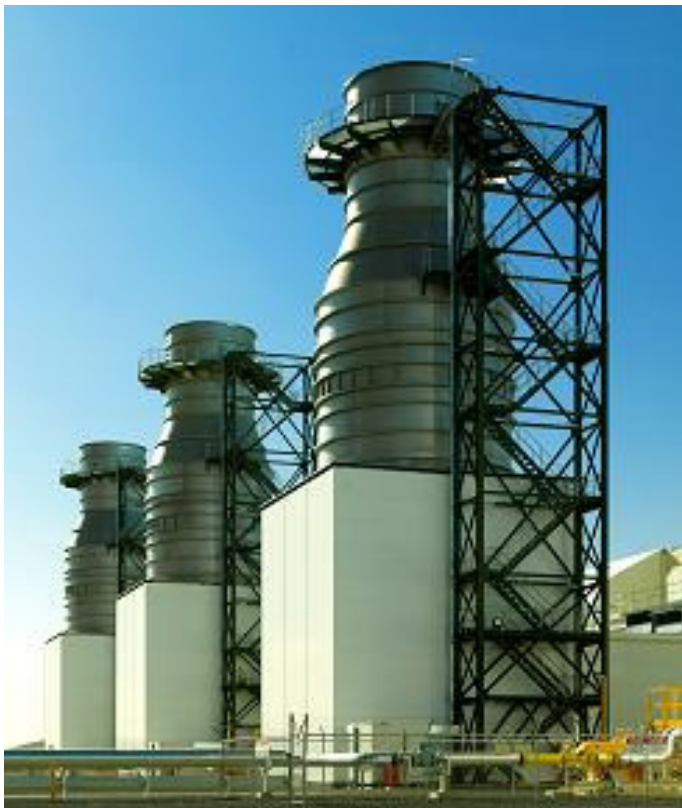
Fig. 5: Stack with few upstream straight stack diameters available
