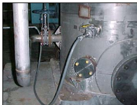
Figure 1: Unsuccessful installation using a traditional insertion sensor mounted in a down flow pipe.
