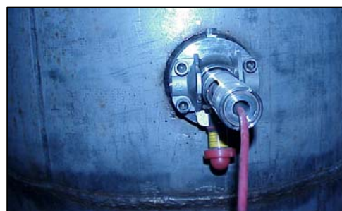
Figure 2: Close up of the TB18 valve welded on the up-flow 12% consistency stockline
