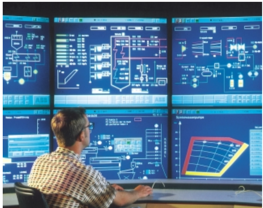
Wall with large-screen display terminals for controlling and monitoring the process 3
