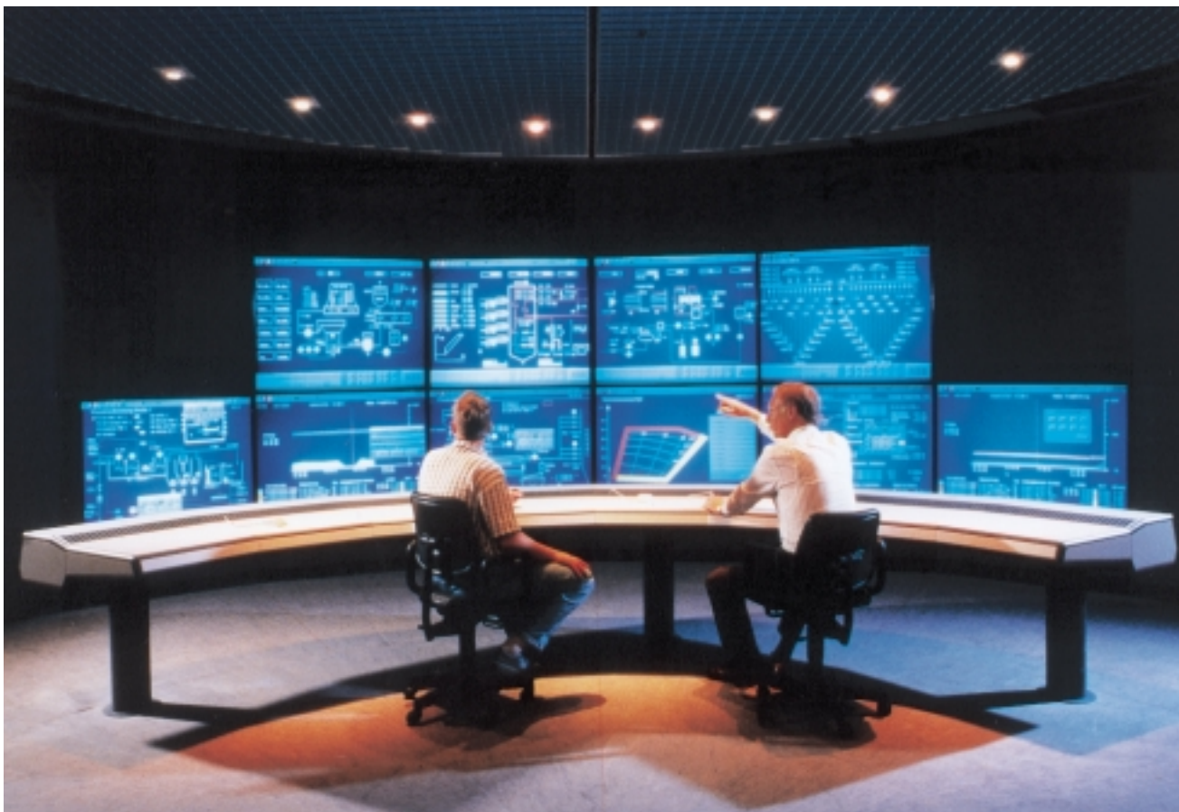
Control room in the 900-MW dual-unit Schkopau power plant
