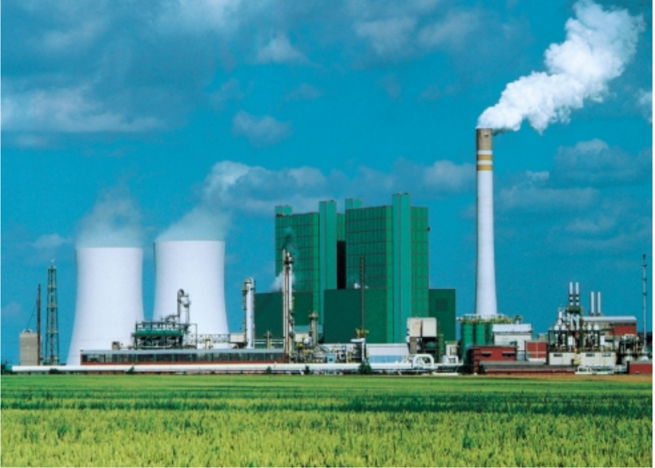
900-MW Schkopau power plant in Germany. The plant's two units, which are fired with brown coal, operate independently of each other and generate electrical energy for the national grid and German Railway. Thermal energy is also supplied to chemical facilities nearby.
