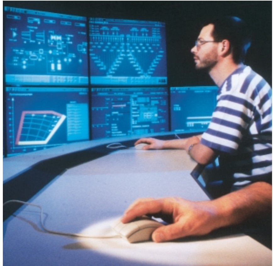
Schkopau power plant is operated exclusively via large-screen display terminals and mouse-controlled interactive communication. 2
