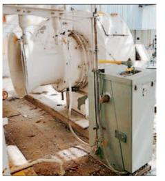
ers, both installed in 1952, are brick-set with forced-draft (FD) intakes and induced-draft (ID) removal fans. Both are rated at 40 klb/hr. The third boiler, a 1965 economizer, has only an FD fan and is rated at 75 klb/hr, though it was typically operated at a maximum of 60 klb/hr.
