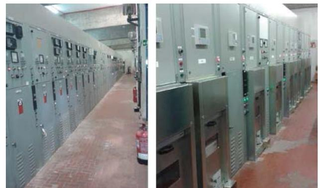
Figure 11. Original switchgear lineup (left) and after retrofill and P&C renewal
