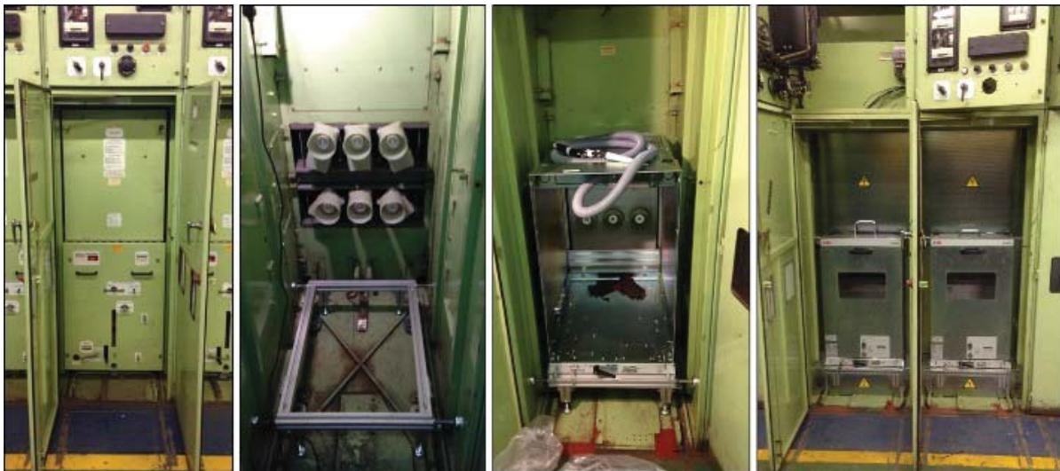
Fig. 5 Retrofill installation sequence
