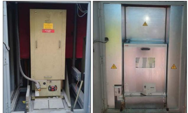
Figure 8. Retrofill of an air magnetic breaker (original at left)
