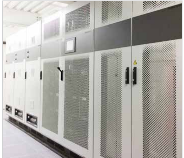
ABB's 1500 kVA PCS100 UPS-I installed at Sensirion in Stäfa
