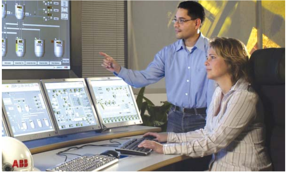
Industrial IT System 800xA Extended Operator Workplace
