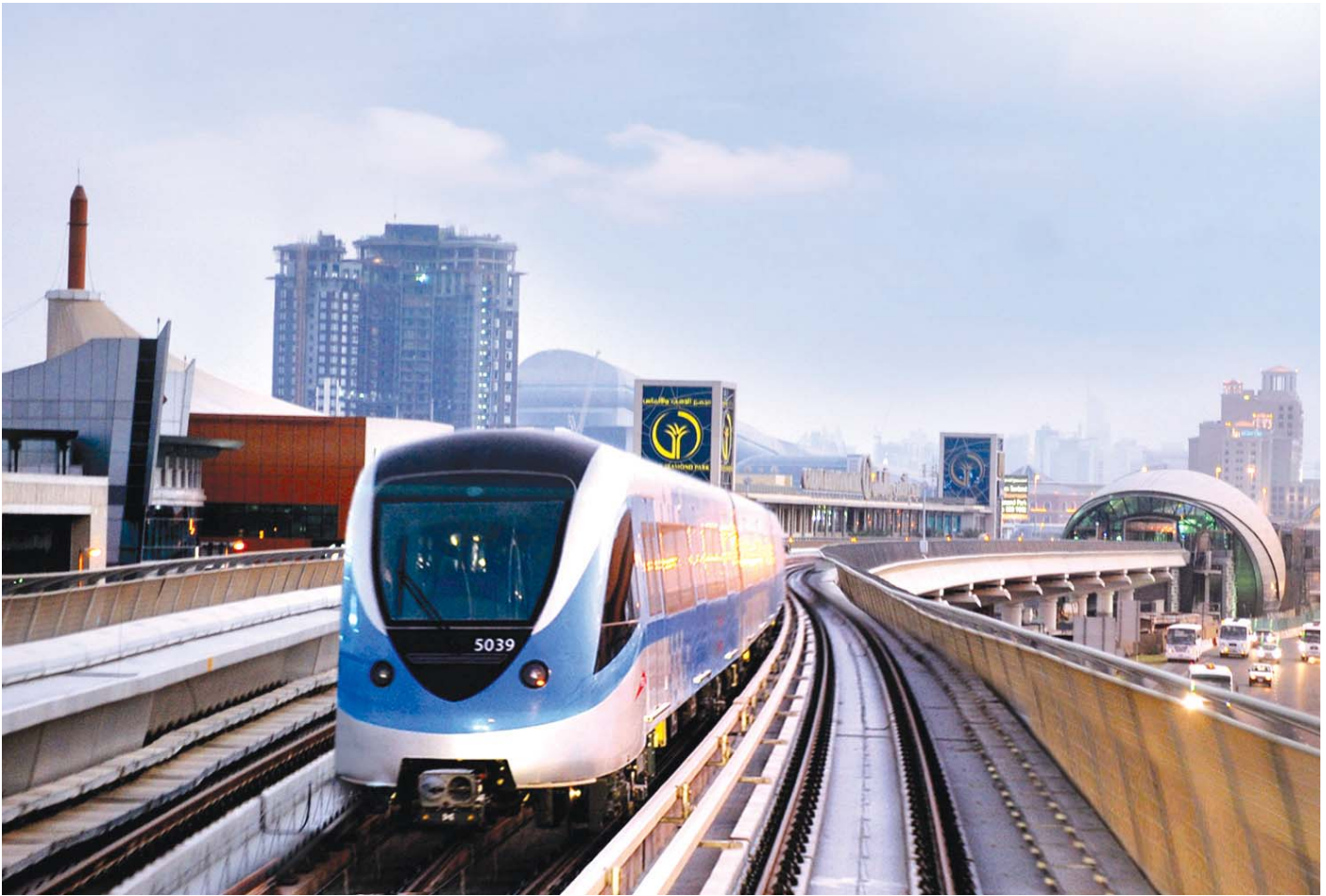
Dubai Metro is powered by ABB substations
