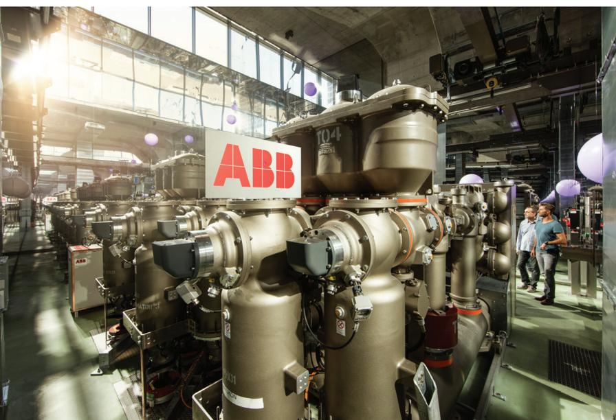
For decades, sulfur hexafluoride (SF<sub>6</sub>) has been the predominant insulation medium for switchgear due to its technical properties. ABB has been developing and deploying alternatives to this greenhouse gas on the path towards greater eco-efficiency and lower environmental impact and is now commissioning the world's first pilot with a new eco-efficient gas mixture.
