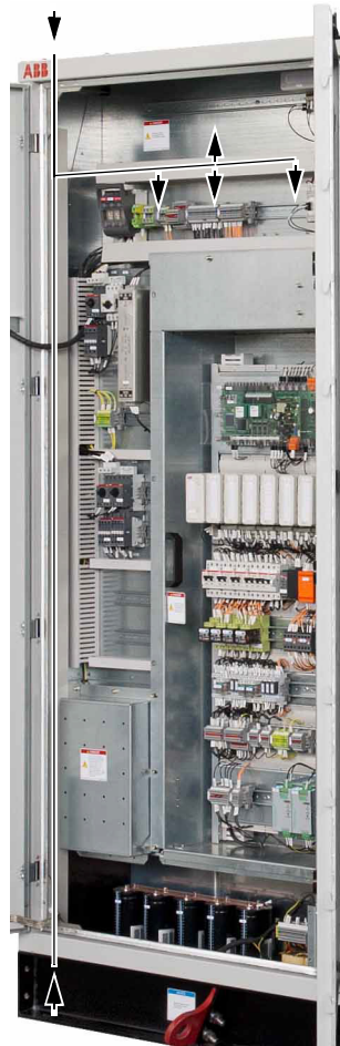
Fig. 6-14 Routing control cables
