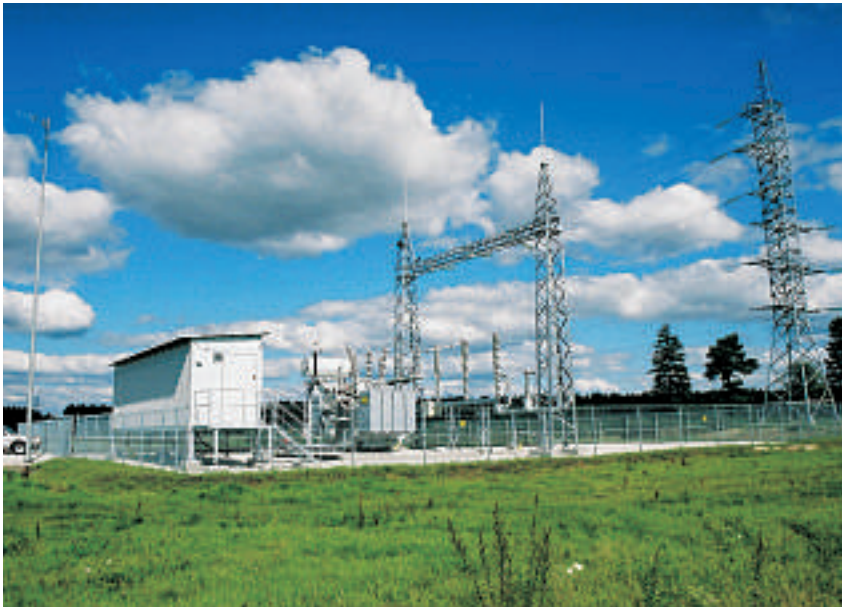
3 PS1 modular substation. ABB has developed a comprehensive product information environment for this substation, comprising a complete Industrial IT based model with all the documentation embedded in a collection of Aspect Objects.
