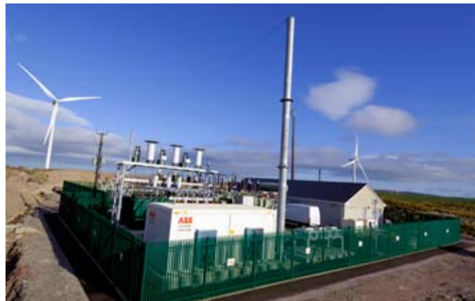
1 x 12.5 MVA PCS 6000 STATCOM for Midas wind farm, Ireland
