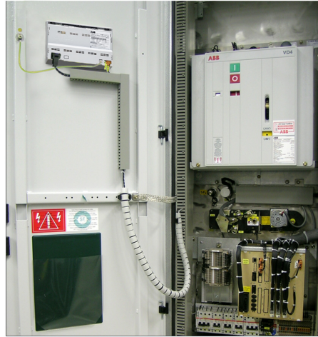
Fig. 4 Mounting of the base unit in the LV compartment and the HMI on the door.
