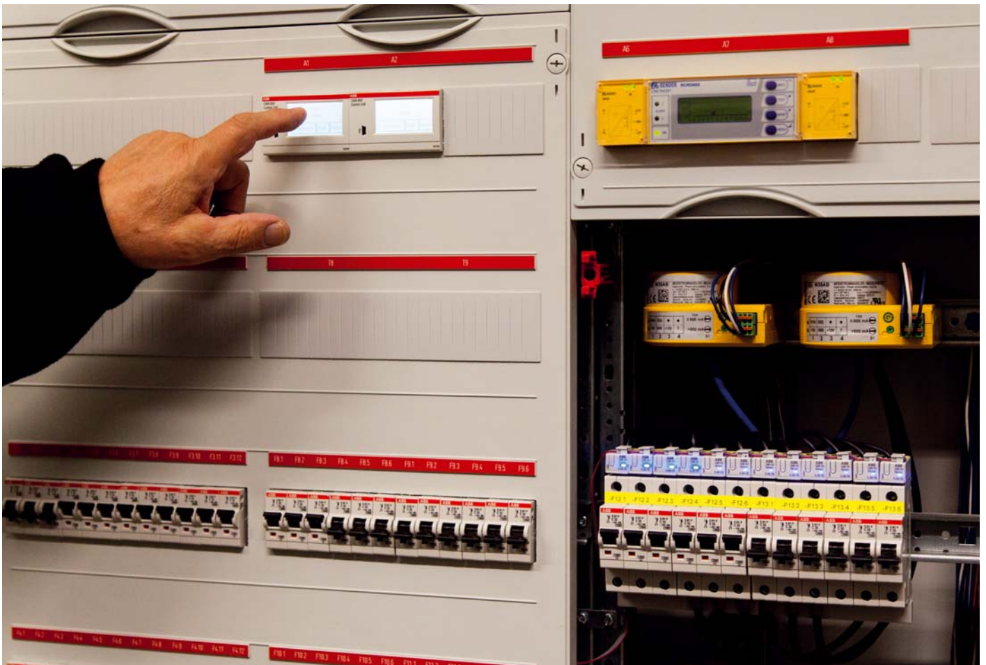
The CMS multi-channel measurement system allows both AC and DC currents to be monitored.
