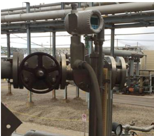
Accurate level measurement of toxic liquid using LMT200 transmitter
