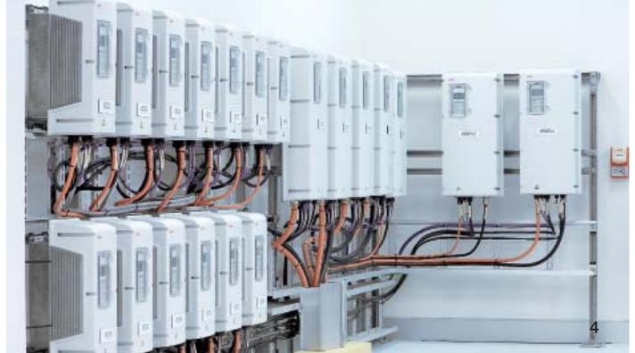
1 AMA motors, powering the energy recovery booster pumps | 2 ACS 1000 variable speed drives controlling the high pressure and energy recovery booster pumps | 3 11 kV vacuum casted (VCC) dry type VSD supply transformers | 4 ACS800 variable speed drives controlling the intake, booster, filter backwash and potable water pumps
