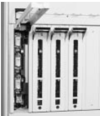
Switch-fuse in the supply cubicle. Due to breaking on both sides fuse replacement always takes place when the unit is dead. The door is interlocked and can only be opened when the switch is in the closed position.
