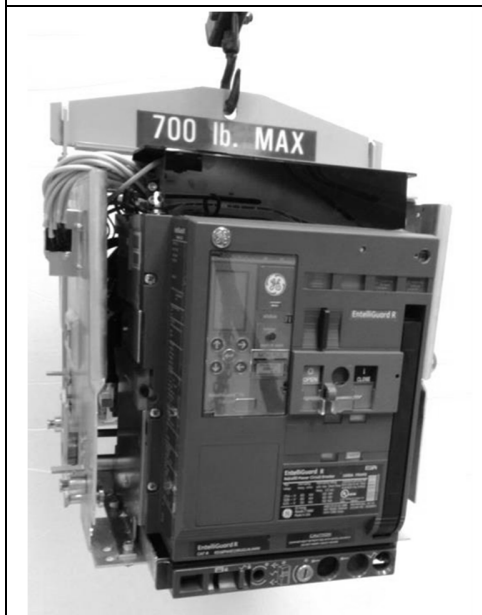
Figure 8. Entellisys Retrofill—Using Lifting bar and hoist
