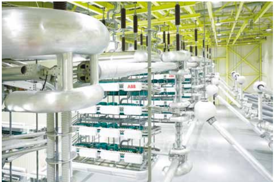
UHVDC valve hall: The thyristor valves of the North East-Agra \pm 800 kV HVDC link to be constructed in India will resemble the one in this picture. The image shows a ultrahigh voltage valve hall of the Xiangjiaba-Shanghai \pm 800 UHVDC link in China, delivered by ABB to State Grid Corporation of China (SGCC)
