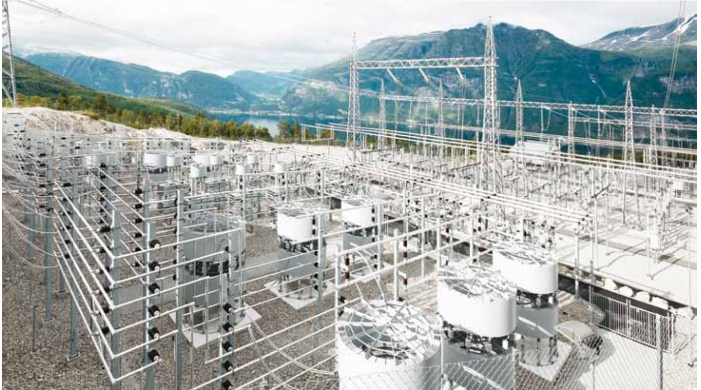
FACTS enhance the capacity, security and flexibility of the power transmission systems
