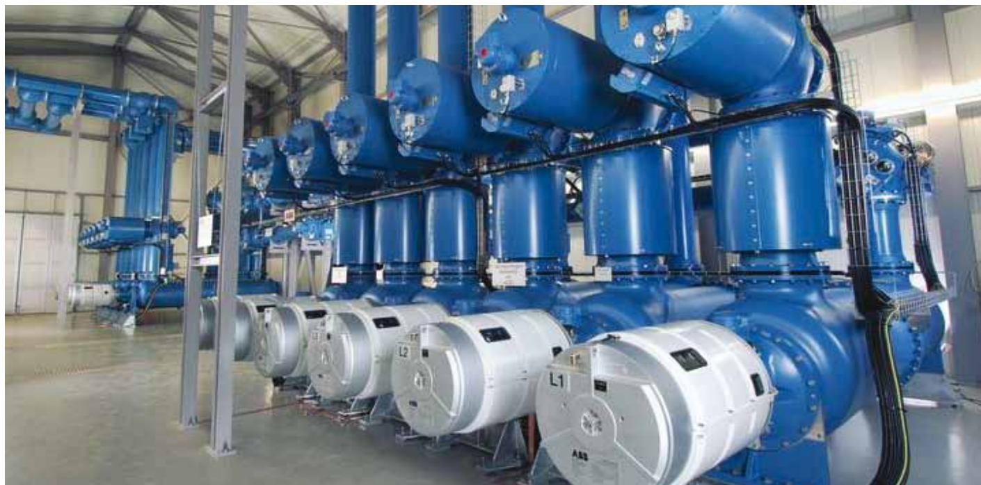
Gas Insulated switchgear helps provide reliable power
