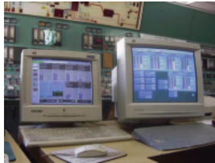
Close-up of both workstations, ABB's Industrial IT (right) emulating FOXBORO's faceplates (left)
