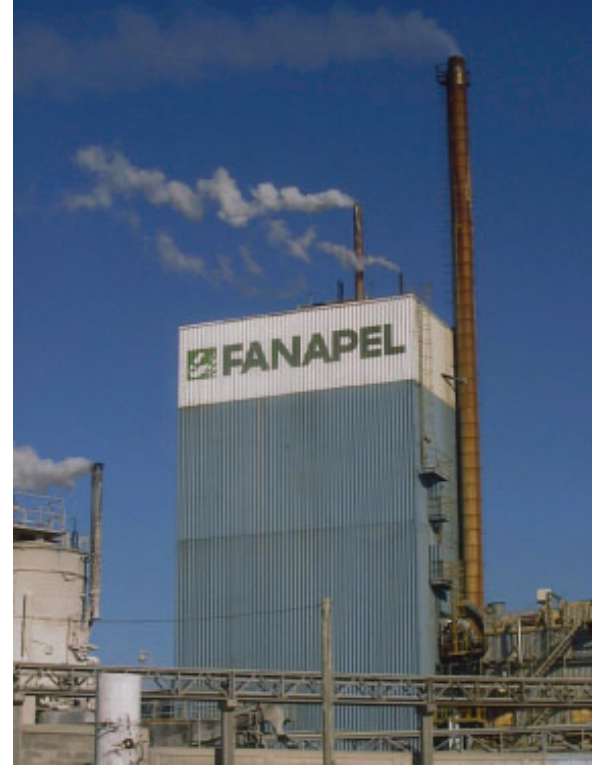
FANAPEL's recovery boiler
