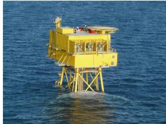
Fig 6. Offshore converter station BorWin alpha offshore Germany evacuates wind-generated power.
