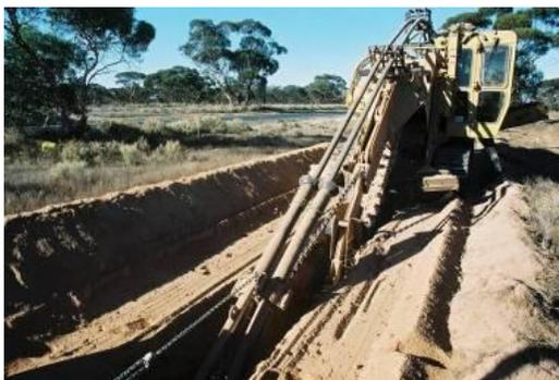
Fig 2. Cable laying in Australia
