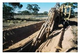
Fig 2. Cable laying in Australia
