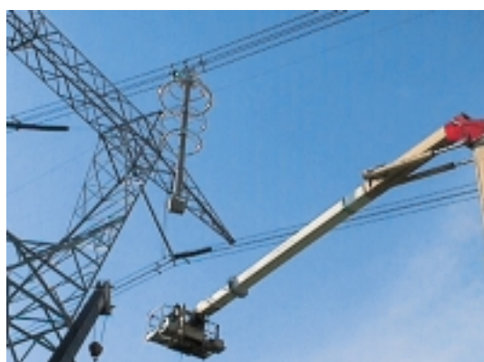
Installing PEXLIM on AEP 800-kV equipment
