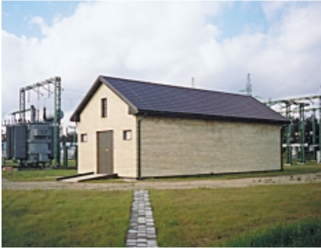
3 One of the substations at Ropazi, Latvia, which ABB equipped with a station automation system. The 110-kV switchgear can be seen in the background.
