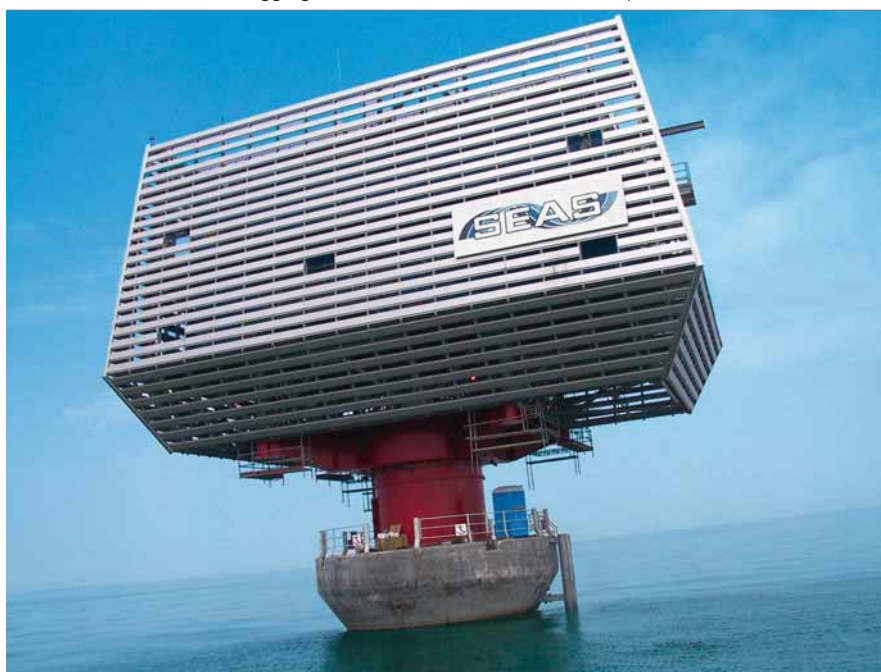
2 Transformer unit for the aggregation of the 72 wind turbines of the park
