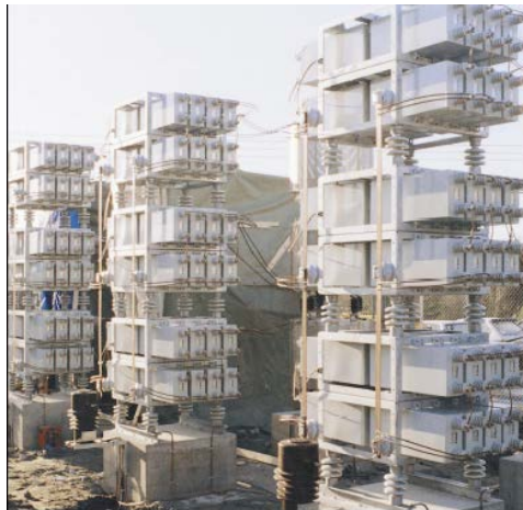
Figure 3.53: Three-phase capacitor bank built out of rack-installed one-phase capacitor units
