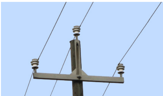
Bare conductor overhead line with normal phase distances
