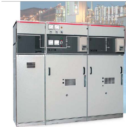
Figure 3.105: A section of typical 24 kV secondary medium-voltage switchgear
