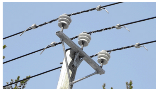
Covered conductor overhead line with reduced phase distances
