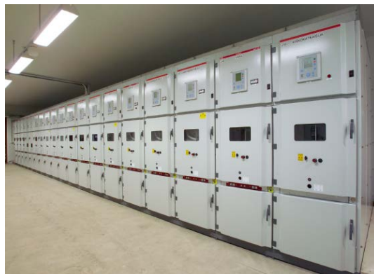
Figure 3.47: Air-insulated primary switchgear equipped with Feeder Terminals
