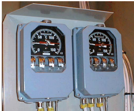
Figure 3.44: Top-oil thermometer and winding thermometer main units fitted on the side of a power transformer
