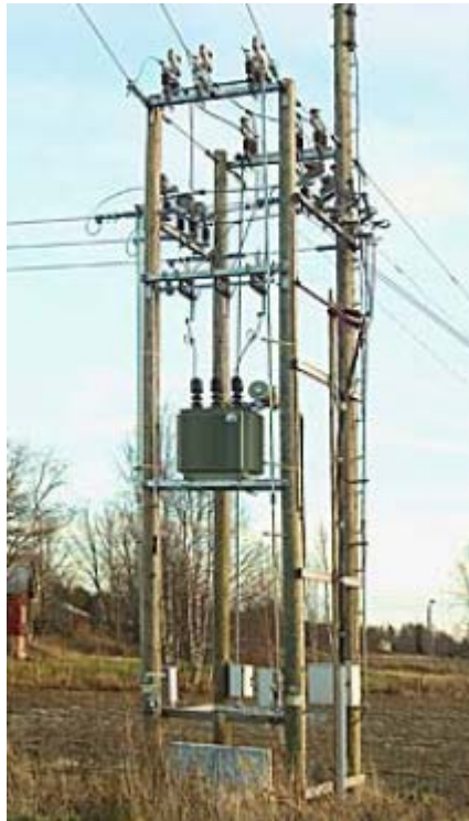
Figure 3.119: Pole-mounted secondary distribution substation
