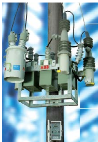
Figure 3.56: A three-phase bank of pole-mounted one-phase capacitor units with voltage measurement, primary load current switching devices and control box
