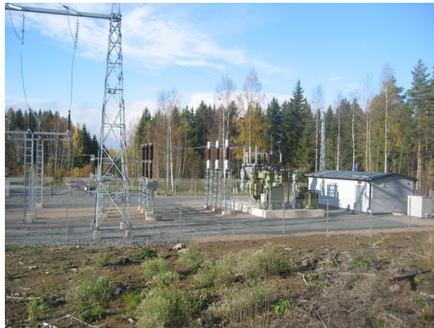
Figure 3.2: A typical rural primary distribution substation 110/20kV
