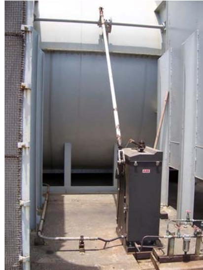
Typical installation of LP Type Linear Pneumatic Actuator on Boiler Over fire Air control.
