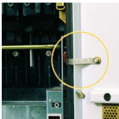
Door earthing system.
