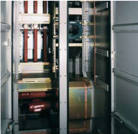
Arc proofing is guaranteed by reinforced doors and a segregated construction.
