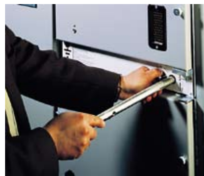
Contactors racking-in with the door closed.
