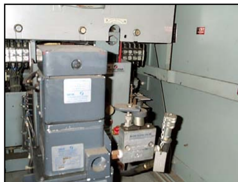
Hydraulic Mechanism
