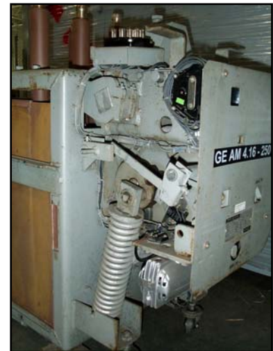
Spring Stored Energy
