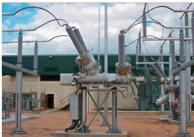
1 ABB'S compact Pass MO 170kV hybrid switchgear combines various functions
