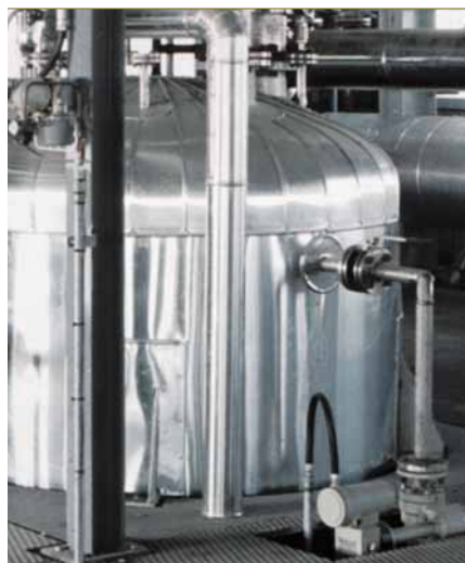
3 Fine chemical plant: Energy optimization methods permit significant cost savings
