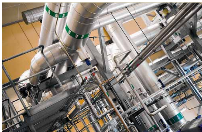
2 A preliminary audit carried out for a European chemicals manufacturer predicted savings equivalent to ten percent of the total site utility costs
