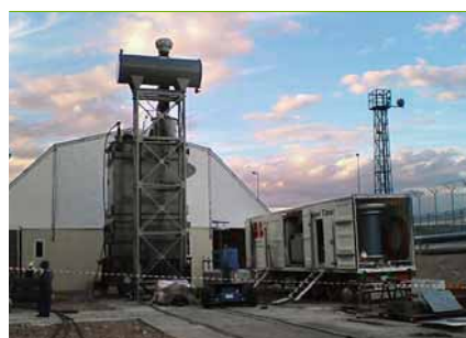
1b A typical set-up for transformer testing at a nuclear power plant
