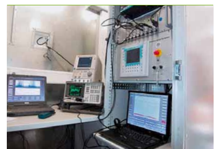
1c Mobile High-Voltage Test System control room
