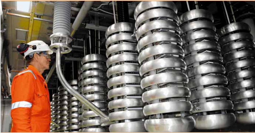
3 IGBT valves – the heart of the converter
