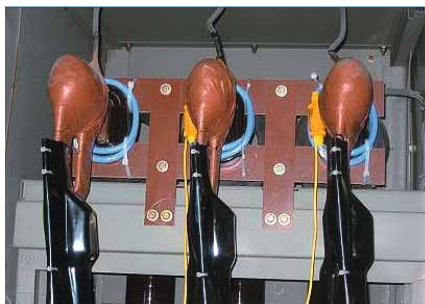
3 Retrofit Rogowski-coil sensors
