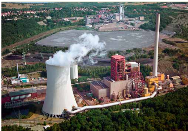
2 The Weiher III power plant, location of the first boiler startup installation
