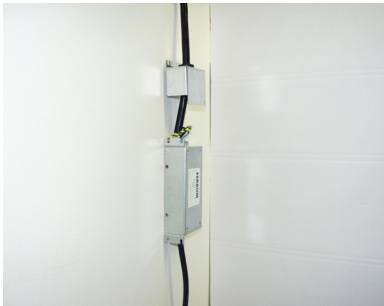
Mounting the assembled unit with RFI-filter
