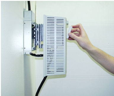
Installing the control panel
