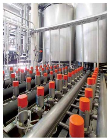
The CIP wash solutions are circulated in the pipelines by centrifugal pressure wash pumps, the speed of which is controlled by ABB machinery drives.
