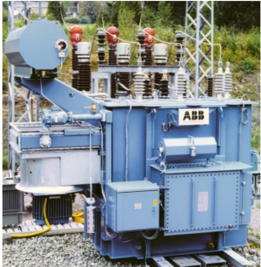
ABB tap-changer, type UZ, mounted on the outside of a transformer tank 3
