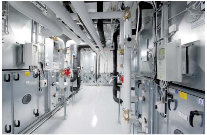
Pumps and fans are controlled via 30, ABB standard drives for HVAC with native BACnet, thus allowing them to be integrated without gateways while being fully visible throughout the system.
