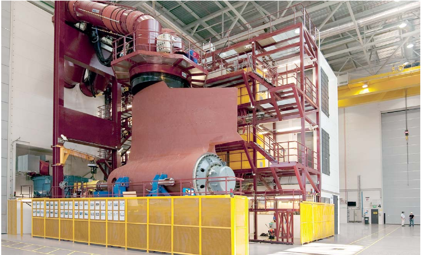
A BACnet-based HVAC system controls air quality while also assisting with functional testing of Azipod marine propulsion units.
