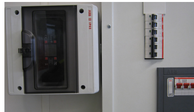
Figure 3: ESP D1/LCD unit mounted in a WBX D8 enclosure, next to a main distribution panel. Note the protector and enclosure are mounted sideways, with the text rotated on the LCD display for normal viewing. For best practice use short connecting leads.
