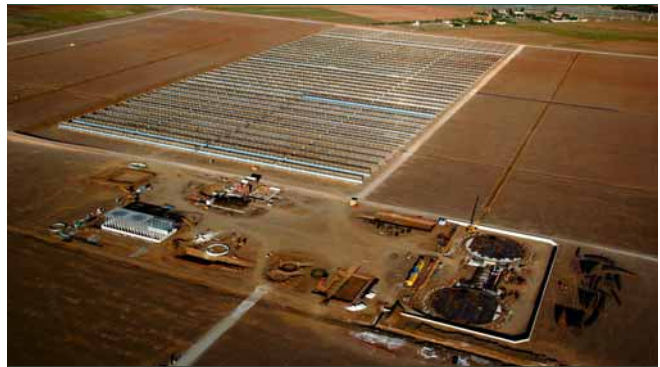
5 Parabolic troughs in fields facing the sun
