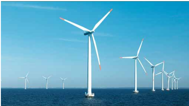
4 Offshore wind turbine connected by ABB submarine cabling
