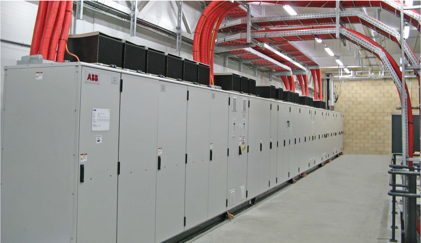
ACS 6000 multidrive, with a total rated power of 36 MVA, controlling the test benches at CENER.
