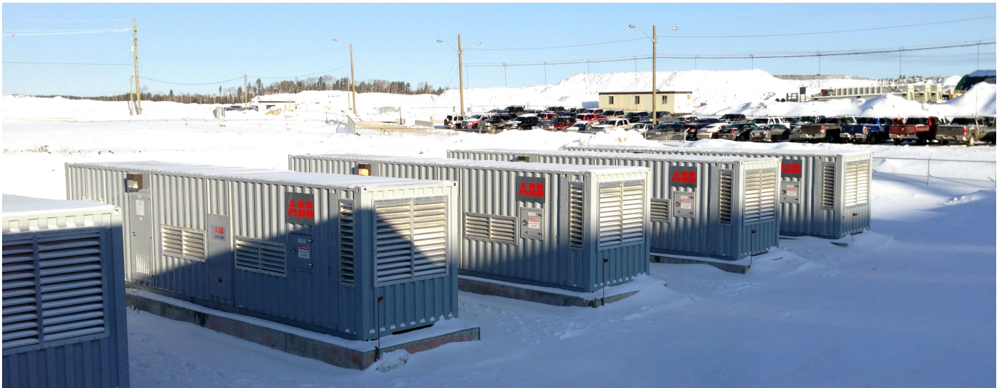
ABB's STATCOMs in operation during Matachewan's winter months.
