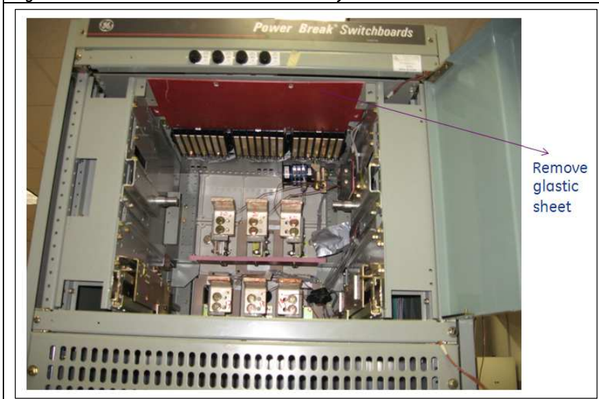
Figure 11. Remove Glastic Sheet – AKR-30S only
