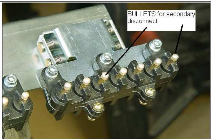
Figure 21. AKD-8—Seven Bullets to a Block, Three Blocks (Exploded View) (Model 1)
