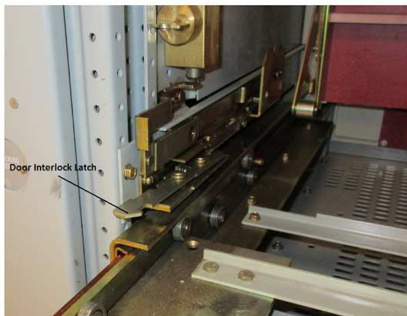
Figure 46. AKD-8 (AKR75/100/125)—Door Interlocking Components
