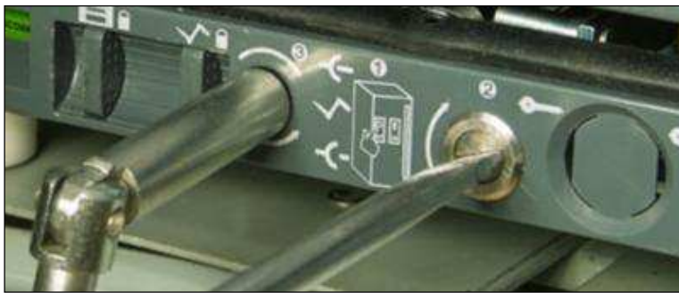
Figure 16. AKD-8—Racking Tool and Screwdriver Inserted
