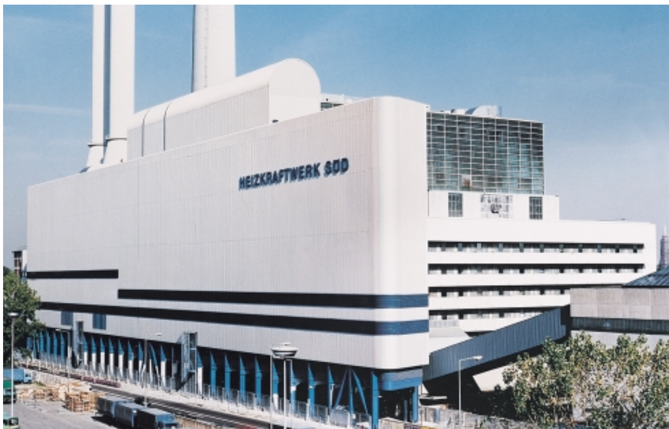
München Süd, Germany's first district heating plant based on waste incineration to be equipped with the SCR denox system 6
