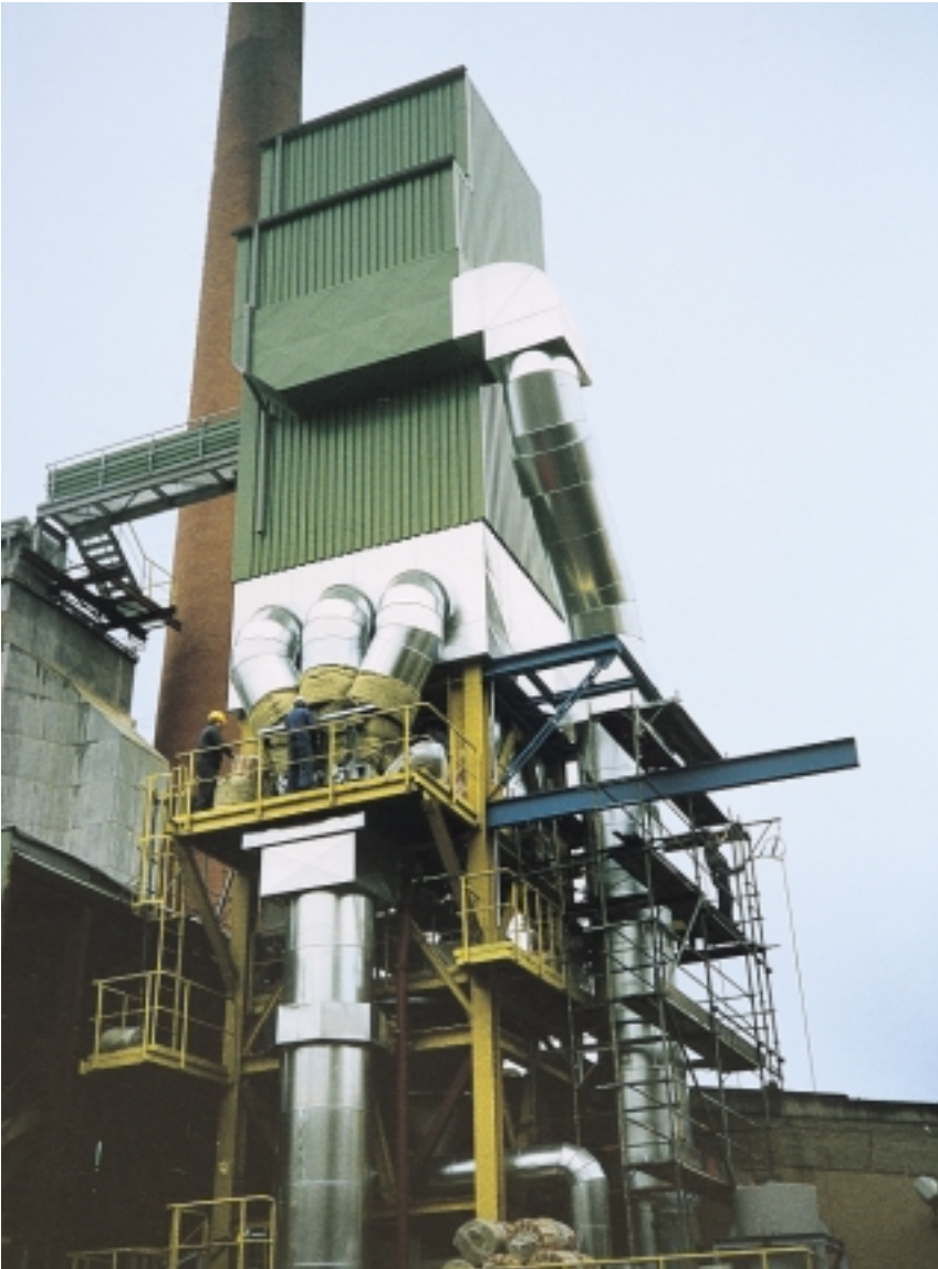
Filsorption stage with scrubber using a sodium hydroxide solution, as retrofitted recently in the waste incineration plant at Zirndorf in Germany 5
