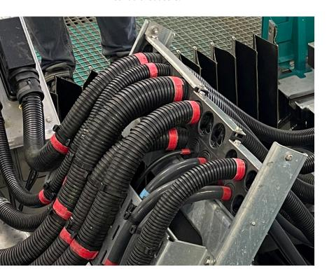
The PMA® TRUST™ modular support system is a lightweight, compact solution with high impact-resistance. Thanks to the new design, external dimensions are reduced to the very minimum and internal spacing between adjoining conduits is very small. Each element can hold different combinations of both conduits and cables in various sizes.
