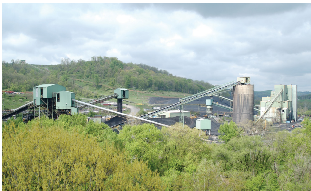
Figure 1. Digital solutions that integrate data and real-time optimisation of processes throughout a mine can help boost productivity and reduce unplanned downtime.
