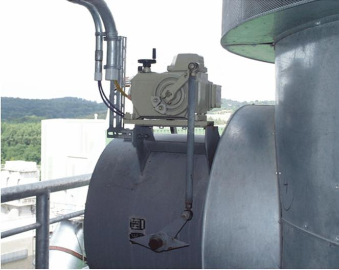
Figure 37: Milling air control; rotary actuator RHD250 (rated torque 250 Nm)
