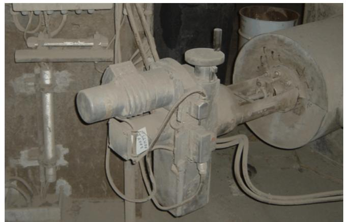
Figure 12: Horizontally mounted linear actuator
