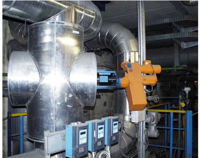
Figure 35: Horizontally installed linear actuator (air control)
