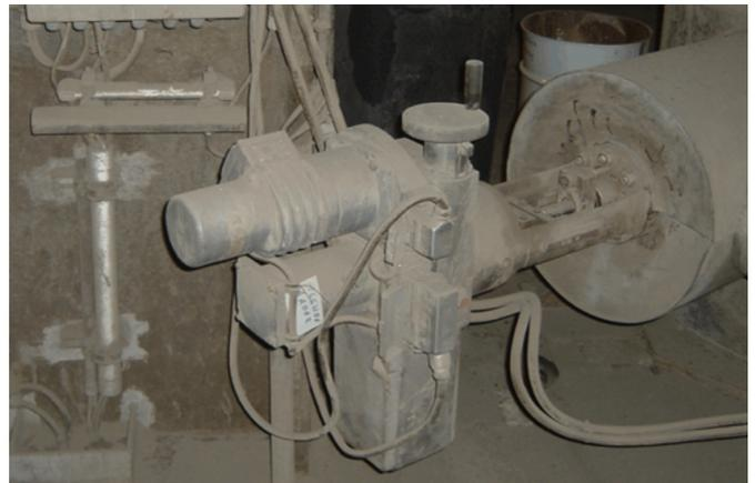
Figure 12: Horizontally mounted linear actuator
