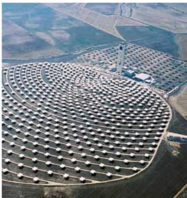
Figure B.8 – Central receiver plant
