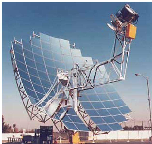
Figure B.6 – Parabolic dish plant
